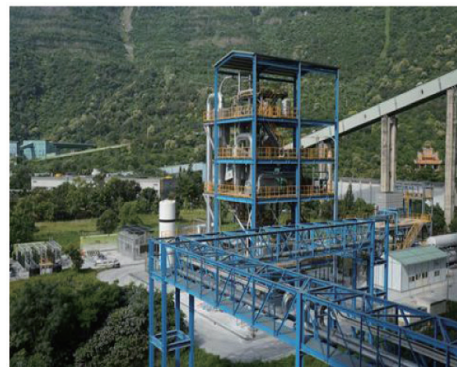
Ind. Tech. Res. Institute (ITRI) & Taiwan Cement Co. Calcium Looping Process (24 t/d)
